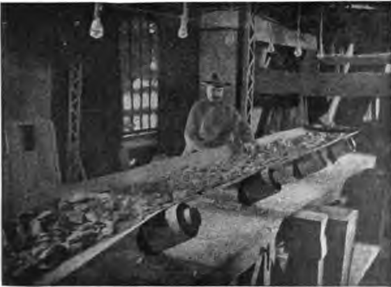
FIG. 10.—ROBINS PICKING-BELT.
